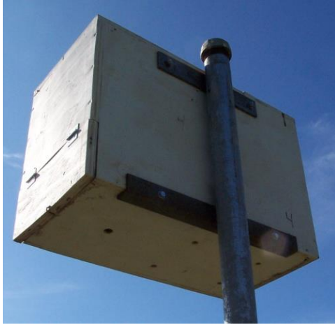
Mounting by welding piece of angle iron
